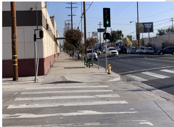
An example of a continental crosswalk
