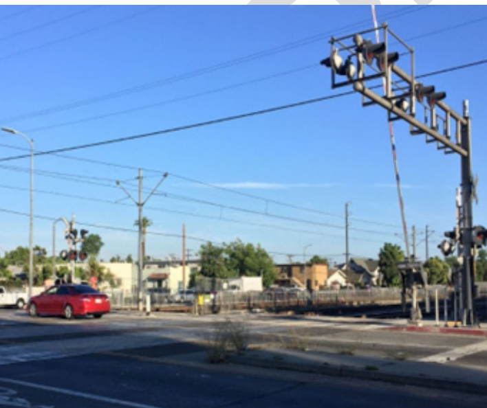
Intersection of 92nd Street and Graham Avenue. Photo Submitted by Yanel Saenz, CAC Member and Florence-Firestone Resident
