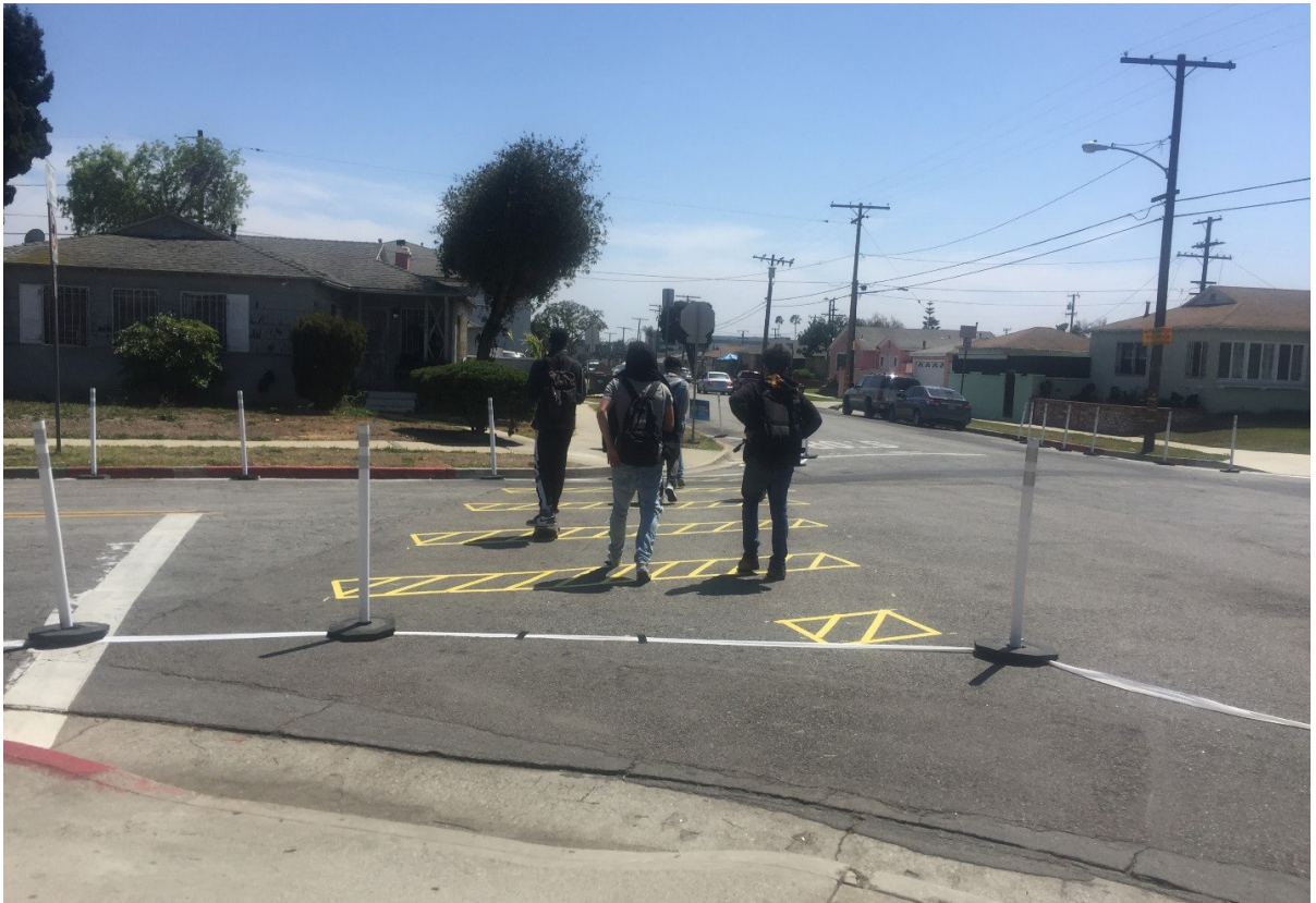
The County demonstrated a roadway reconfiguration, bulb outs, and high-visibility crosswalks in Westmont/West Athens
