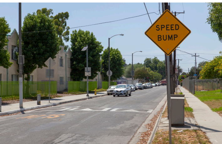
A typical speed hump, supplemented with speed hump signage and pavement markings
