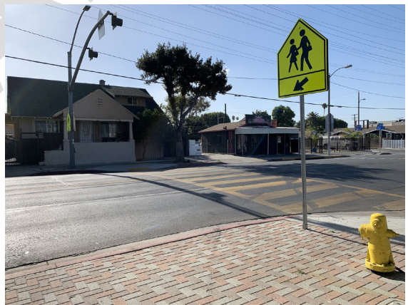
An example of a ladder crosswalk with pedestrian signage.
