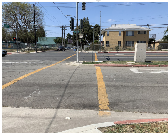
A standard crosswalk with two parallel yellow lines in a school zone on 120th Street
